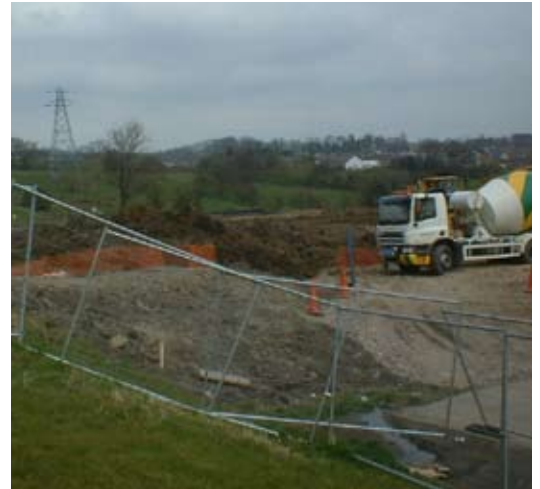
Phase 1 of Riverside Business Park
