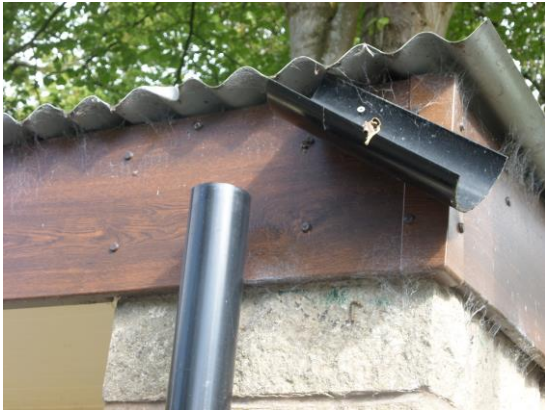
Broken Troughing
